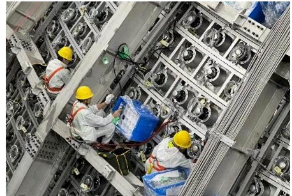
PMT and electronics installation ongoing!
