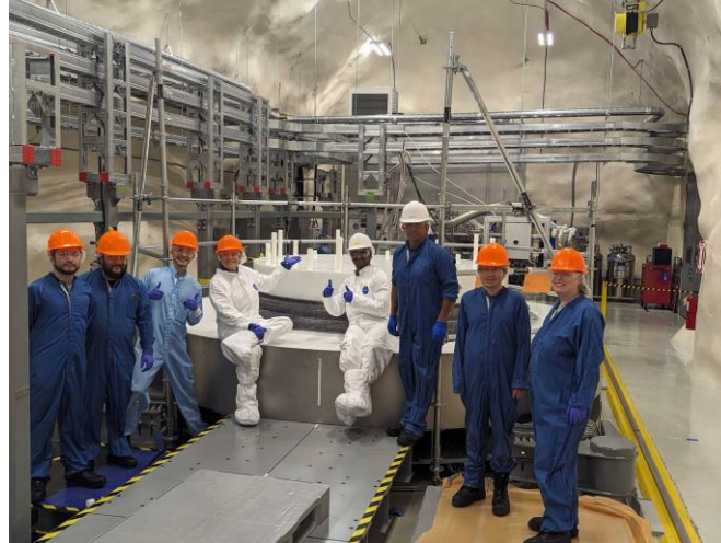
✓ Shield base installation 2023
