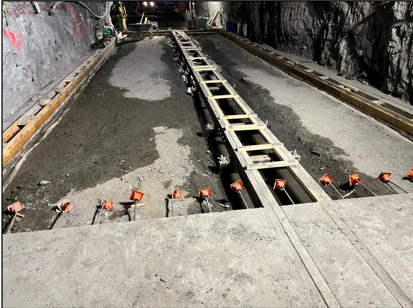
4850-02 Drift Formwork Including Rail
