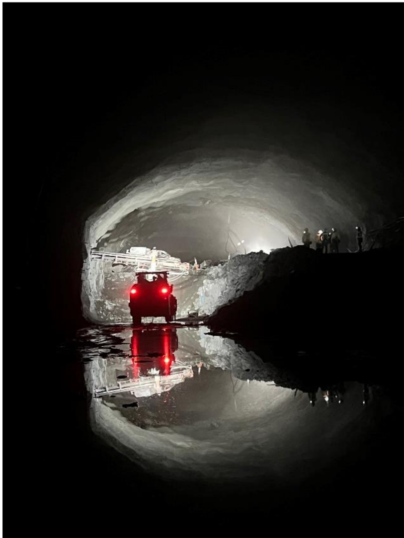
CUC (4850-36) Installing CT Bolts
