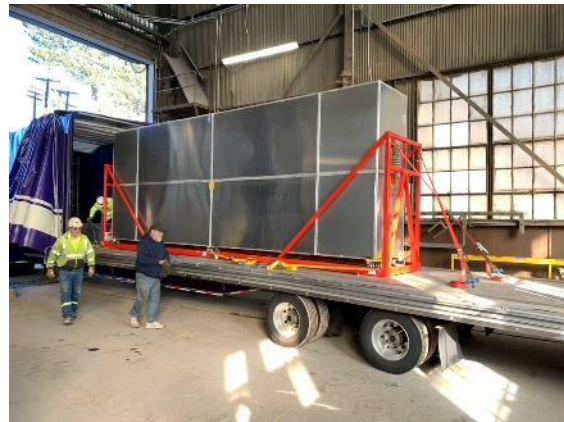
Offload at Crusher Bldg. SURF
