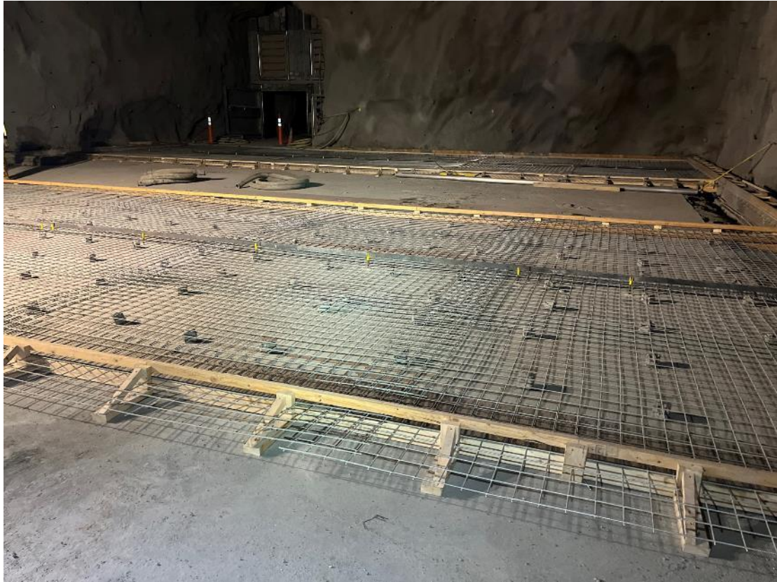
Formwork for 1 st slab section - Central Utility Cavern (4850-36)
