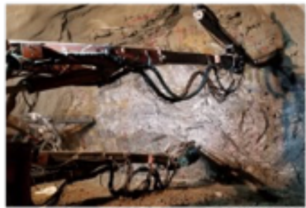
1. Drill Blast Holes
