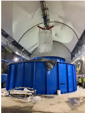
FIGURE 6: The acrylic vessel of OSIRIS being lifted into the steel tank.
