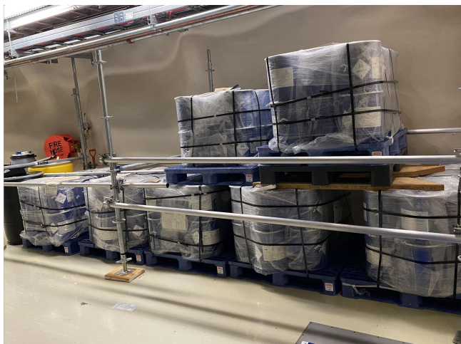
TeA underground storage
