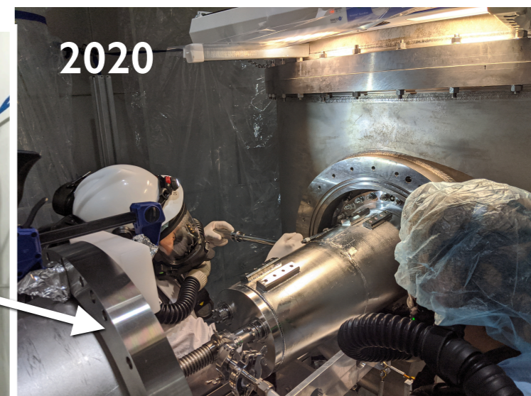
Making up cathode connections (under N2 purge)
