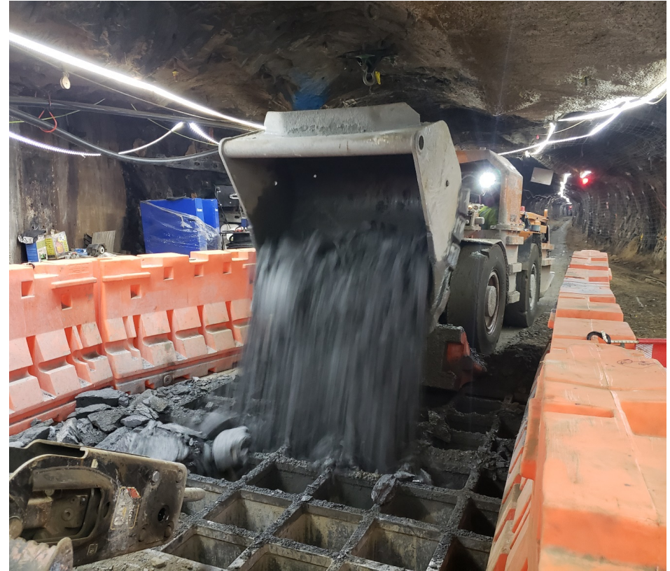
Moving muck and dumping through grizzly into ore pass to be loaded on skips to move to surface
