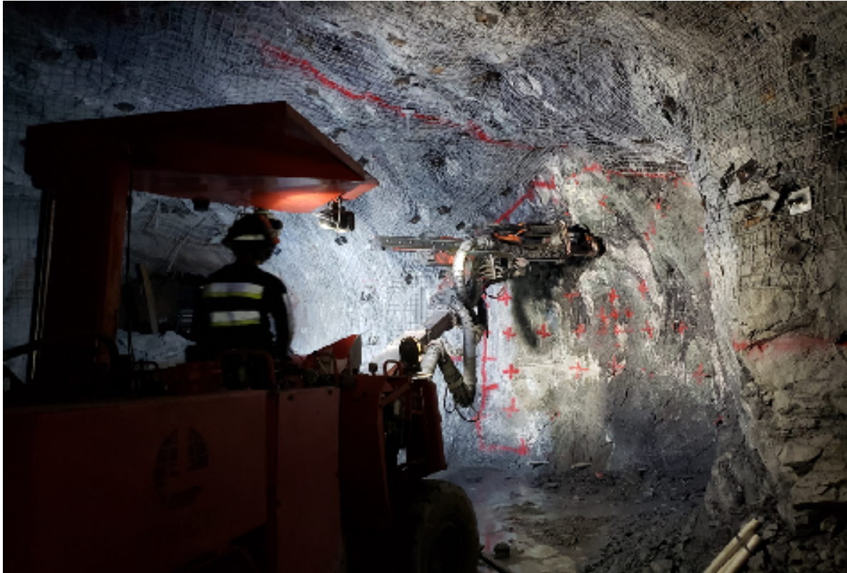
TMI Drilling Blast Holes with Single Boom Jumbo
