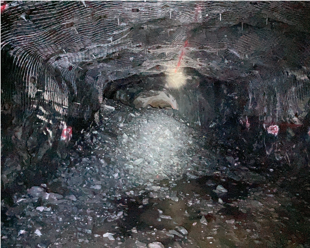
Muck pile, post blast, for electrical substation cavern
